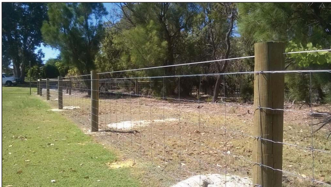
Plate 1: Example of installed conservation area fencing
